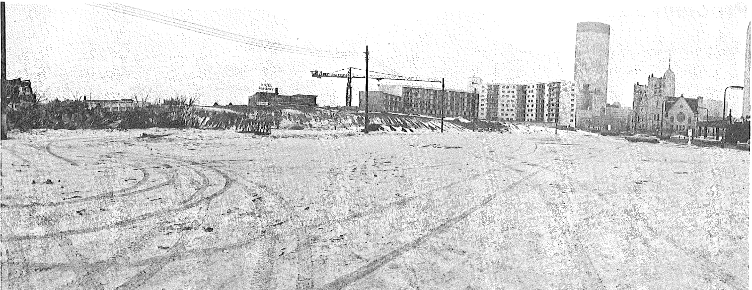
A vast expanse of cleared land (above) awaits redevelopment in the Loring Redevelopment district. At right: Sign promising 201 apartments.
