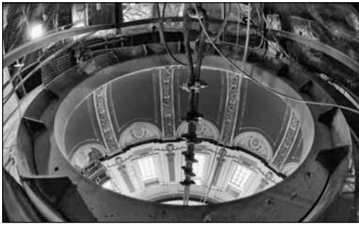
A metal ring has been installed in the top of the dome to allow hot air to rise into the frost dome. The hot air will then be mixed with cool air and exhausted out of the frost dome to outside the Capitol.
