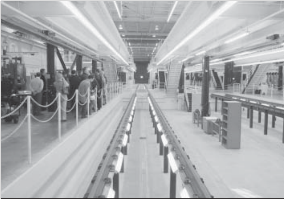
The House Transportation Finance Committee tours the maintenance operations center for the Hiawatha Light-Rail Transit project Feb. 4. Scheduled to begin operation in April 2004, the system will travel nearly 12 miles between downtown Minneapolis and the Mall of America.
