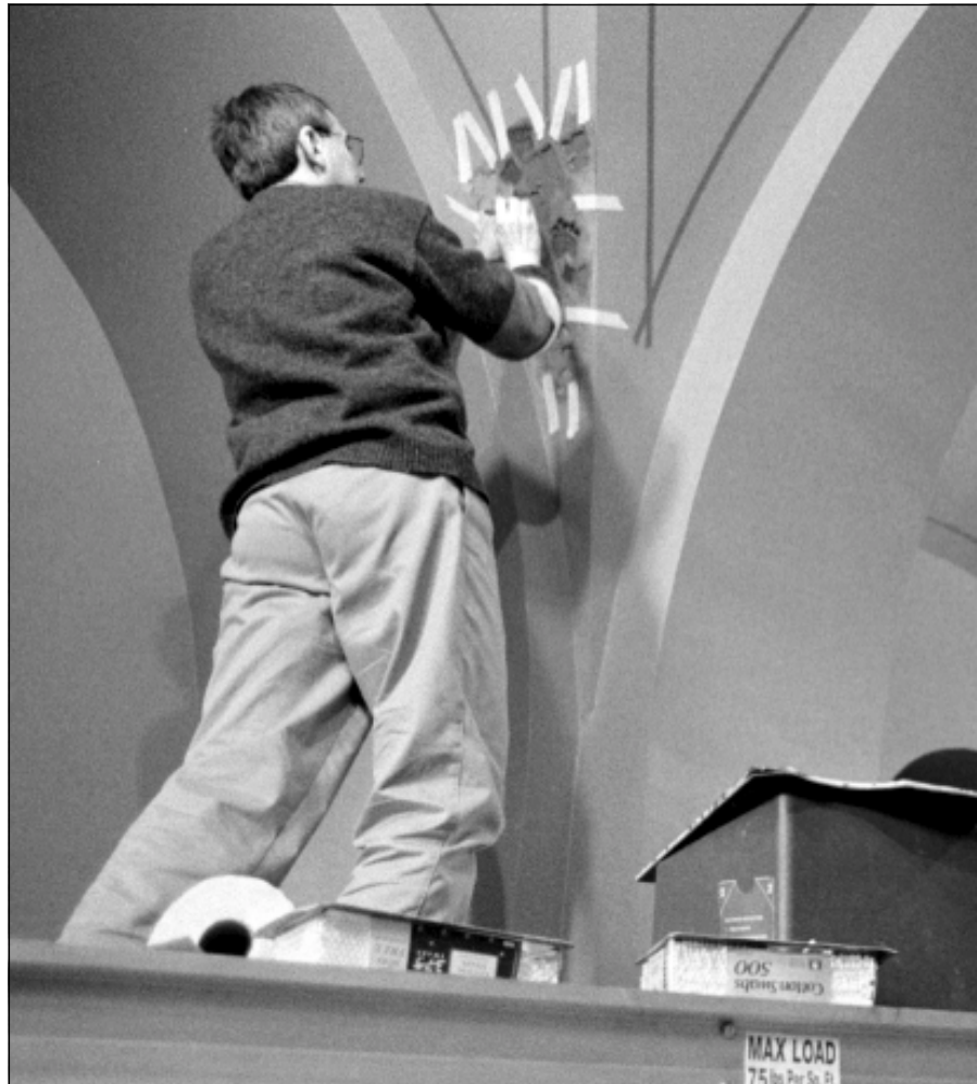
Dan Tarnoveanu, who is supervising the restoration, applies the base layer of paint to a stencil.
