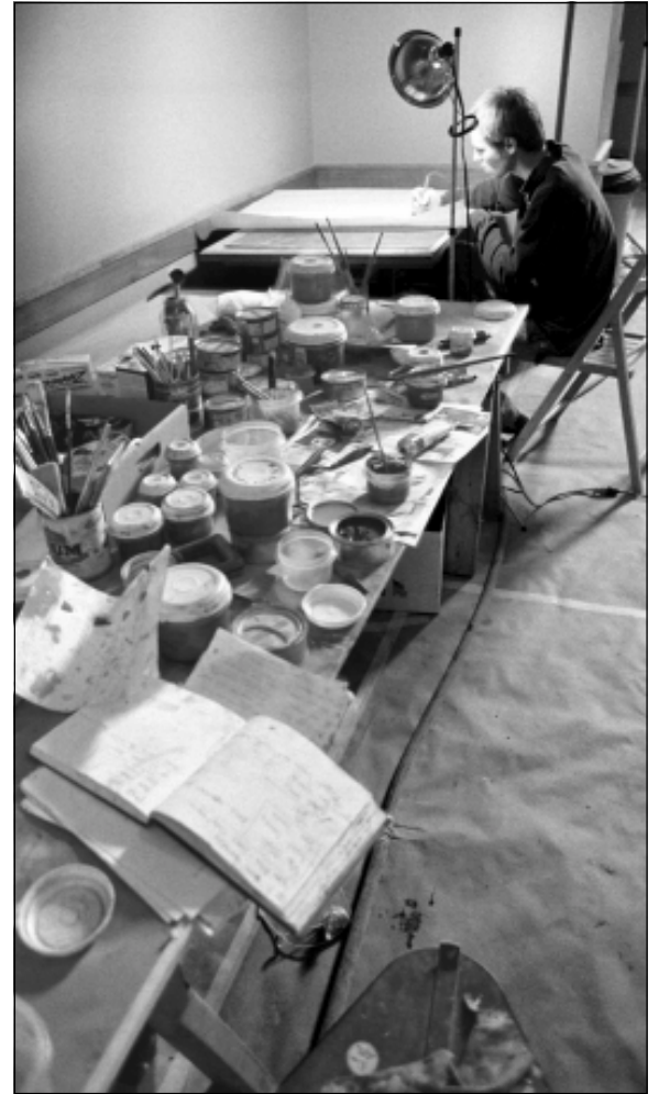
Mike Slagle, an intern from the College of Visual Arts in St. Paul, punches outline holes in a stencil as part of his duties during the restoration of the Capitol cafeteria. Slagle also mixes all of the paints used to restore the stencils on the ceilings and walls.
