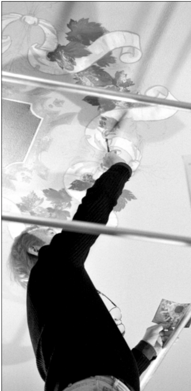
Herman Krumholz applies a layer of paint to the cartouche stencil in the center of the cafeteria's ceiling.
