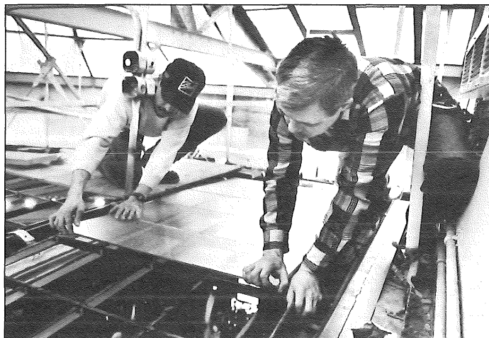
Right: Glaziers fit a large sheet of glass into the skylight's metal framework.
