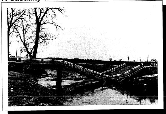
The bridge over Middle Branch of Rush River on CSAH 9 in Sibley County was washed out in April as flood waters moved through the area.
