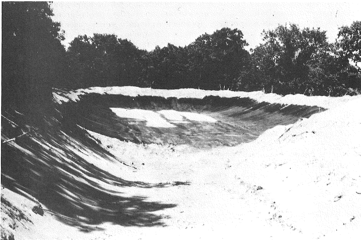
Physical containment measures for disposal sites may include use of liners to protect ground water supplies.
