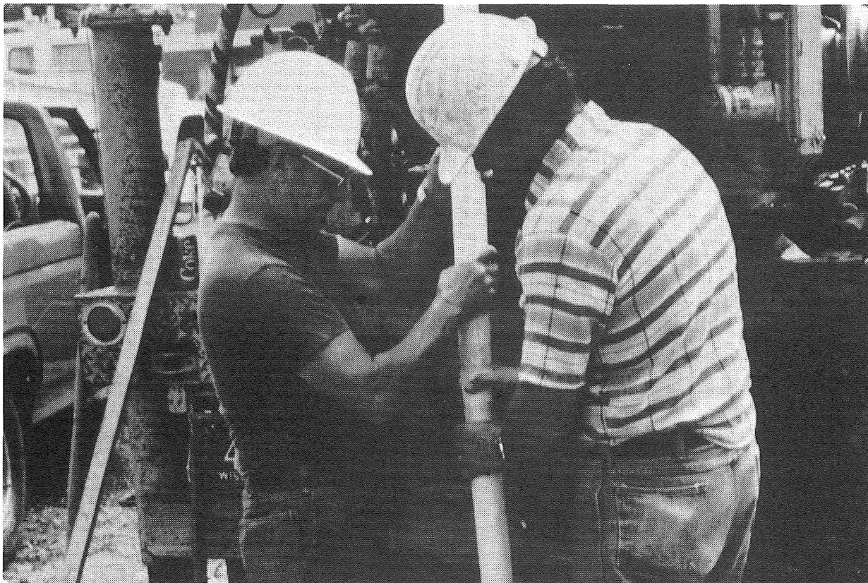
Wells in Minnesota must meet specifications of the Water Well Construction Code, administered by the Minnesota Department of Health (MDH); here, drillers install a plastic-cased well for monitoring shallow ground water near a waste disposal facility.
