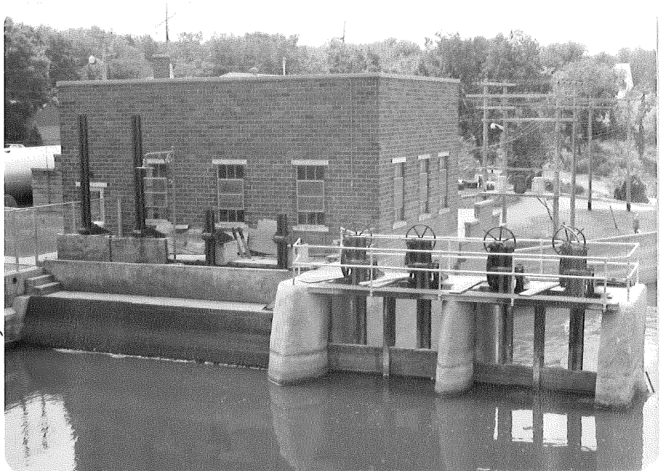
Photo 6. Power house and gate structure at left abutment of dam.
