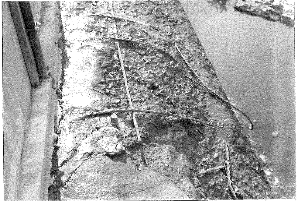
Photo 5. View of right spillway crest showing exposed aggregate and reinforcing bars.
