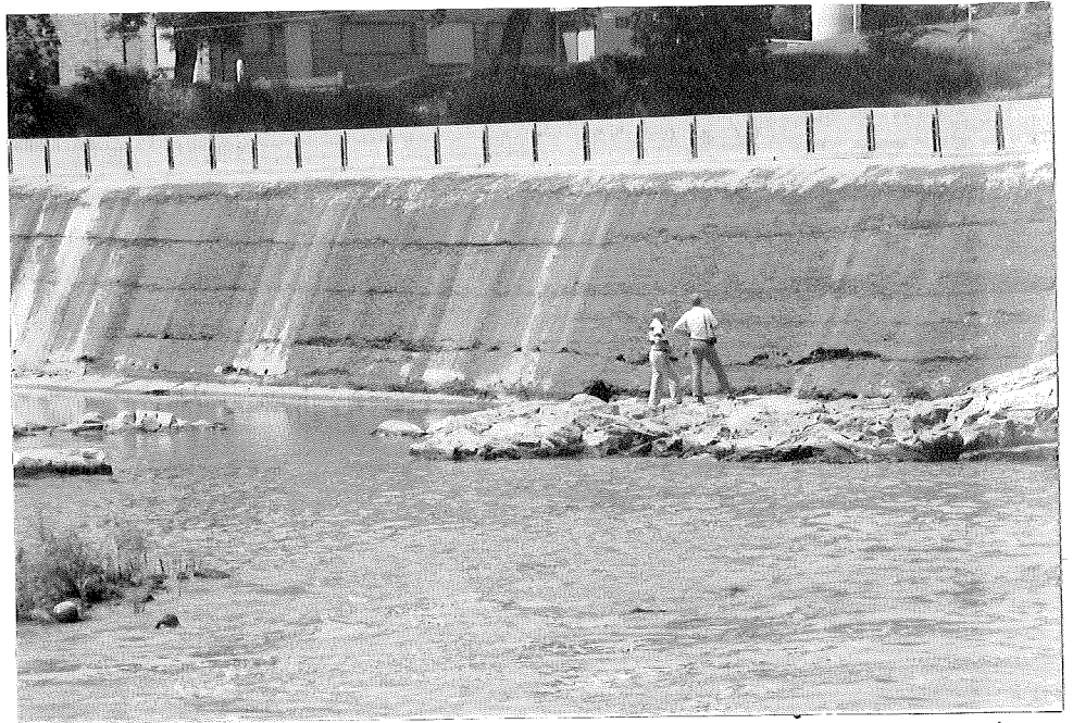
Photo 3. Right downstream face of dam showing cold joints and wood flash boards in place on dam crest.
