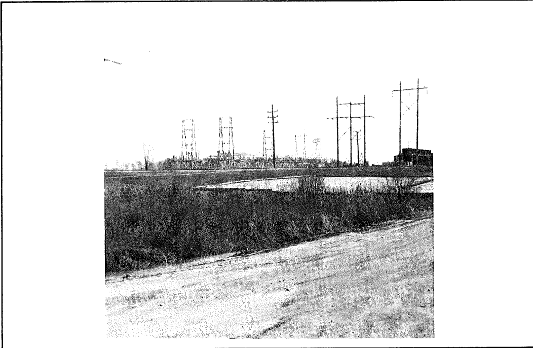
SWITCHYARD AND UNIT 3 COOLING TOWER FROM MINNESOTA T.H. 6 CLAY BOSWELL STEAM ELECTRIC STATION VIEW POINT 2 ON FIGURE IV-116
