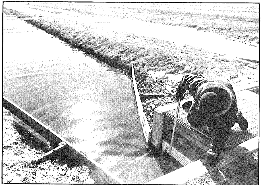
Shyne cleaning an outlet in one of the heated channels.
