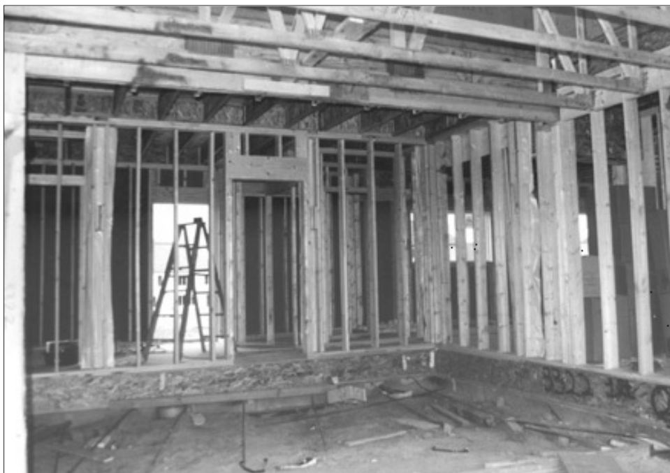
The state building code dictates how housing is constructed or remodeled.
