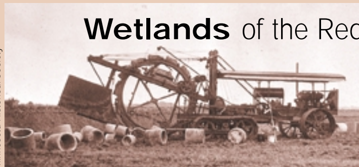
Installing drain tile in the Red River Valley, 1918.
