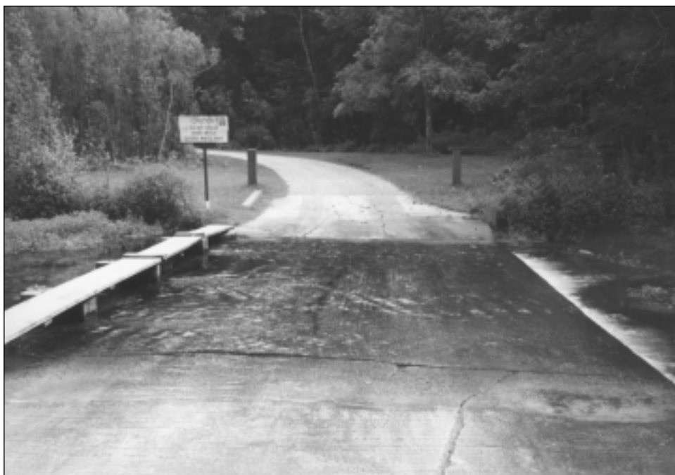
Replacement of the low-water crossing at Beaver Creek Valley is number 22 on the park capital improvement project list.
