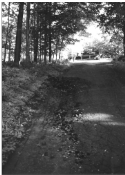
There are some signs of deterioration, such as eroded or flooded trails, in some parks.
