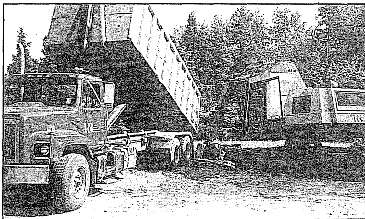
The demolition crew filling in a basement after demolishing and removing a dilapidated building near Floodwood.
