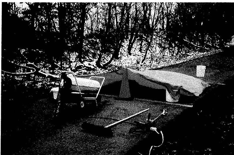
Figure 4. Pavement drying and heating.
