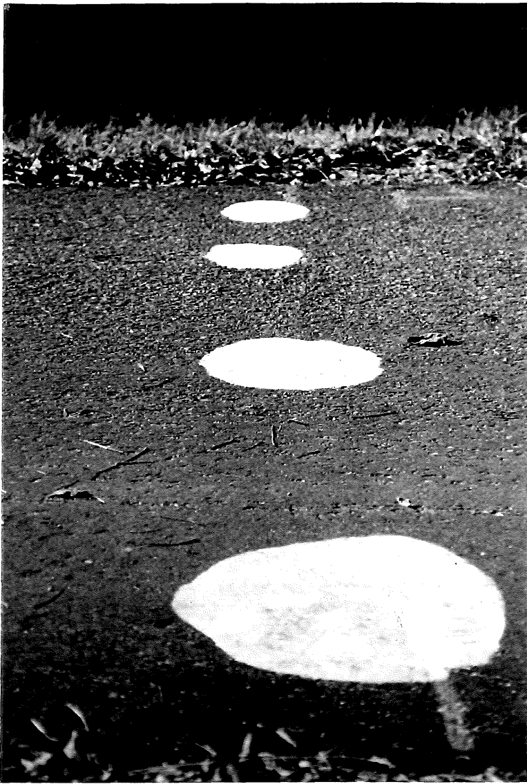
Segment 1 (19East, Type 41A): This segment showed considerable abrasion and loss of aggregate on the south half of the trail, which would probably be the acceleration lane for snowmobiles that have crossed the intersection. The northern half of the trail is not as heavily damaged.
