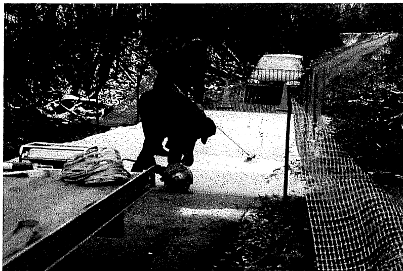
Figure 8. Saw cutting of boundaries.
