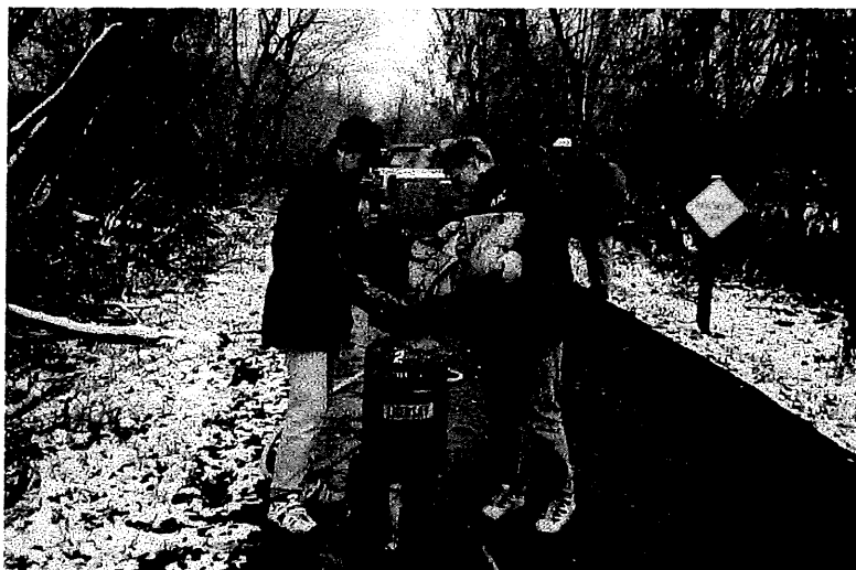
Figure 3. Sandblasting the surface.
