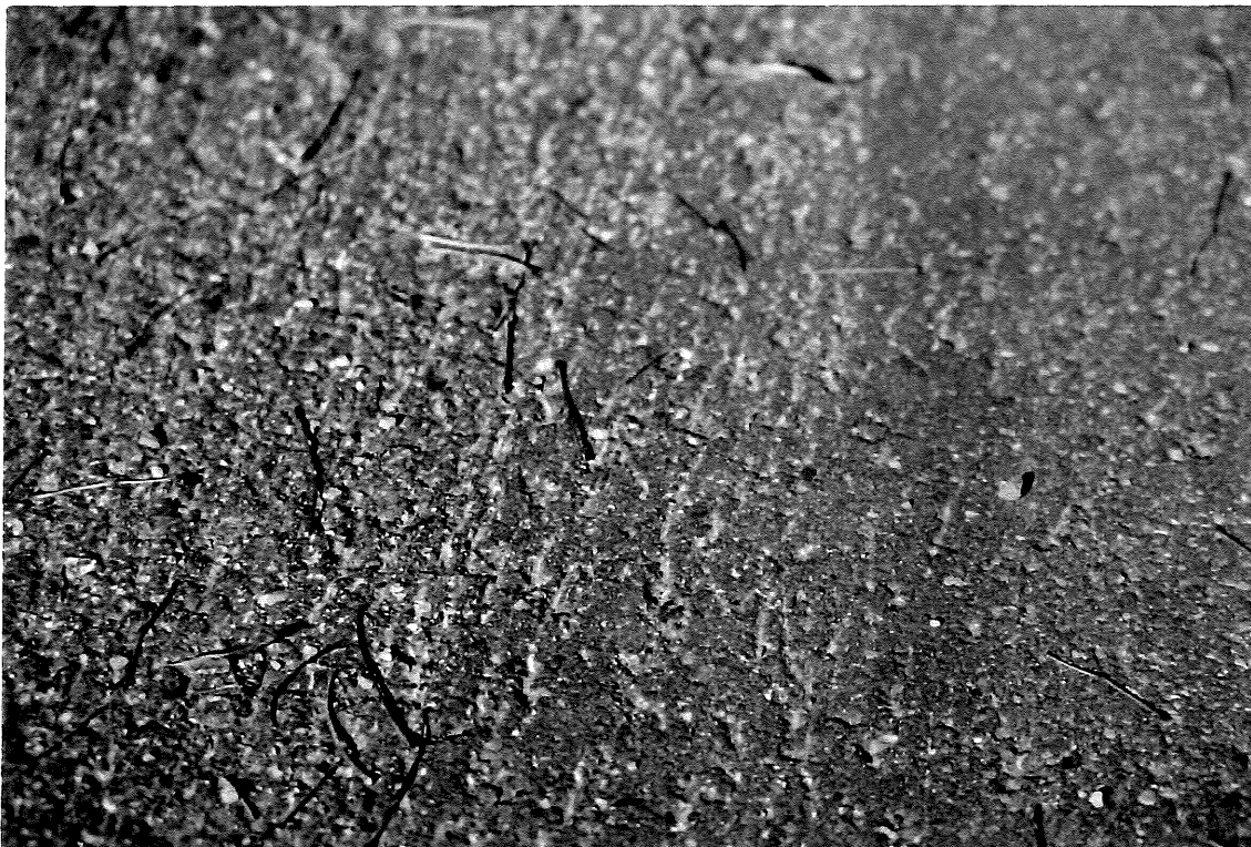
Segment 1 (19East, Type 41A): This segment showed considerable abrasion and loss of aggregate on the south half of the trail, which would probably be the acceleration lane for snowmobiles that have crossed the intersection. The northern half of the trail is not as heavily damaged.
