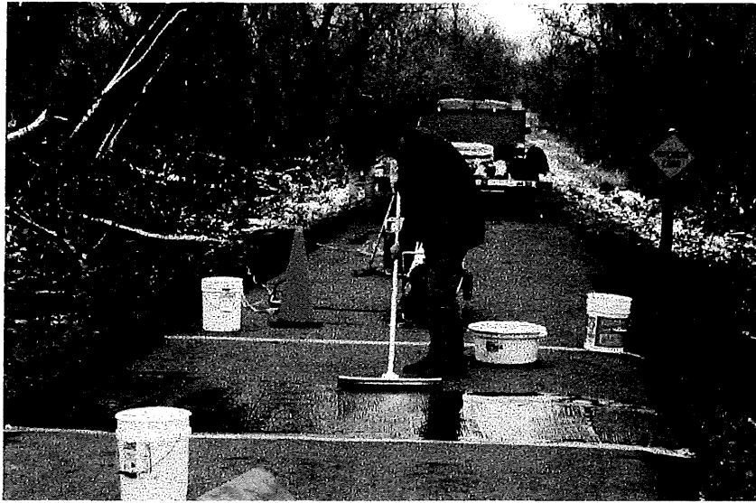
Figure 6. Coating application.
