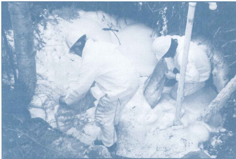
Workers cap an abandoned mine shaft using polyurethane foam.
