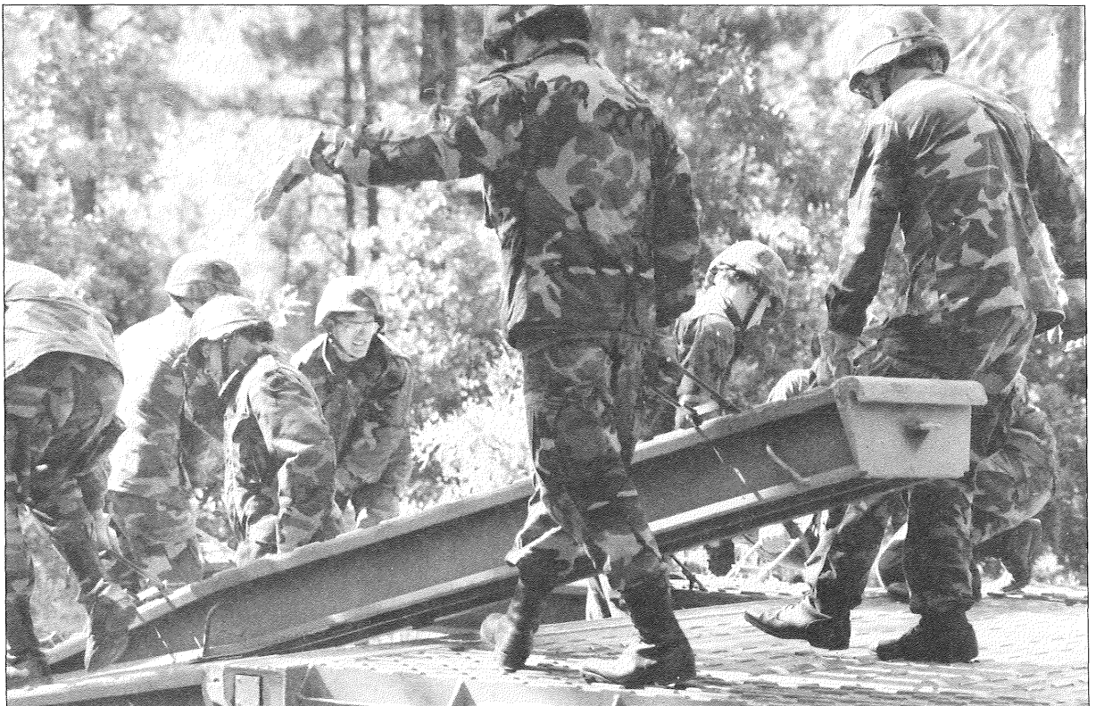
Members of the 682nd Engineers carry medium girder beams to build a bridge at their annual training.
