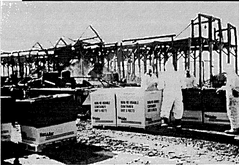
A fire at the Brown County Agricultural Service in Sleepy Eye required a quick response. Although the responsible party paid for cleanup, this is the type of site where MERLA funds may be needed in the future.
