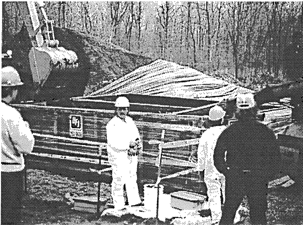
Lead-contaminated soil removal was completed in FY 94 at the McGuire Wire and Salvage Site near Mora.
