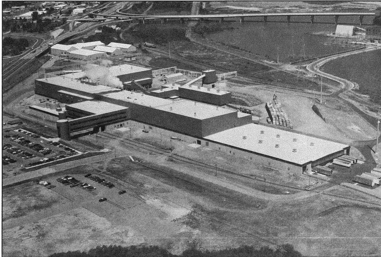
Right: New $400 million Lake Superior Paper Industries plant - Duluth.
