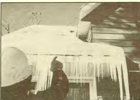
Weatherization Program crews work on mobile homes, blow insulation in attics, teach energy conservation measures and help prevent ice dam build-up on roofs.
