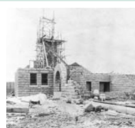
State Reformatory under construction in 1895.
