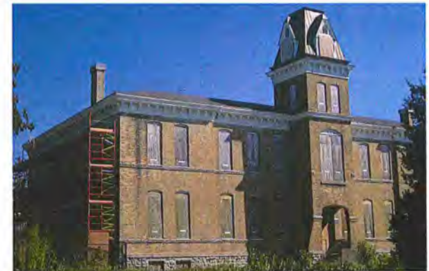
View of Building 67 – Post Headquarters today. All windows were covered in plywood and entry points were secured in 2008. Masonry repairs were initiated in 2010.
