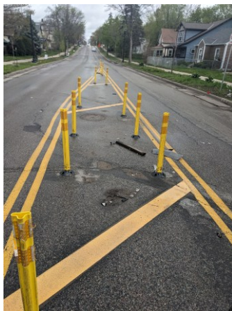
Figure 5.1 Temporary refuge section with bollards and paint.
