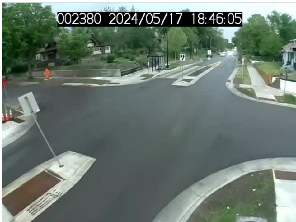
Images of 34 th & Lyndale , pre-installation (top image) and post-installation (bottom image).
