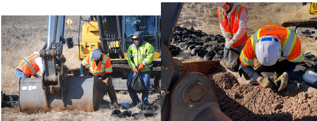
Figure 4.19 Treatment bag removal.
