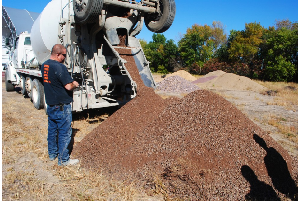
Figure 4.2 Delivery of mixed treatment media.
