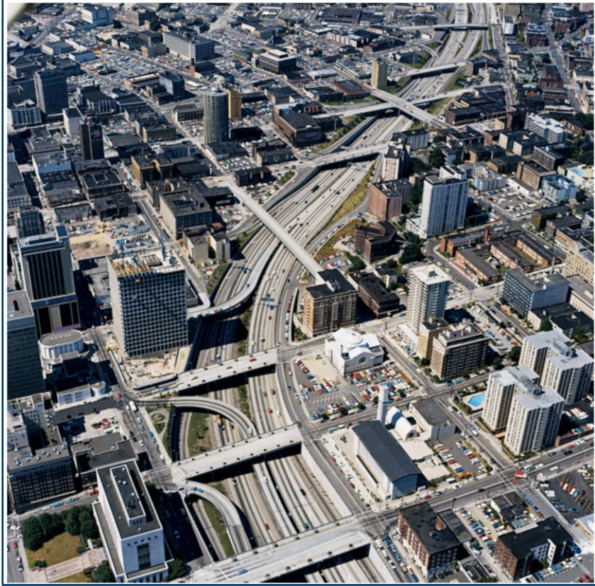
Panel A. Aerial of I-5 before the construction of Freeway Park
