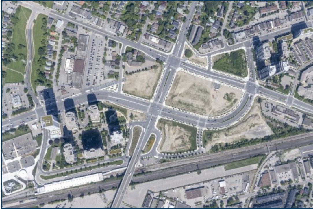
Panel A. Aerial of the area after construction
