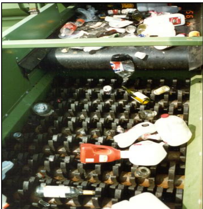
Figure 18: Lubo Fines Screen
