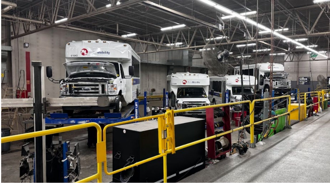
Figure 7-4 Maintenance bays at Transdev’s East Zone facility.
