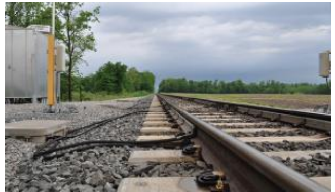
Figure 5: An Example of a Wheel Impact Load Detector
