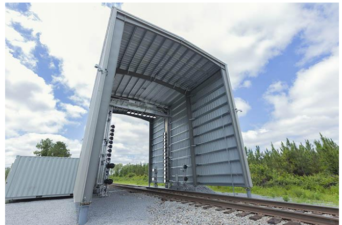
Figure 19: Duos Technology Railcar Inspection Portal
