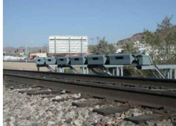
Figure 6: An Example of a TADS Acoustic Bearing Detector site
