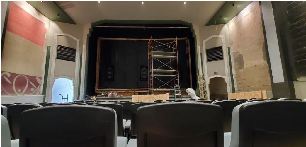
Figure 1: Interior of the Falls Theatre during rehabilitation
