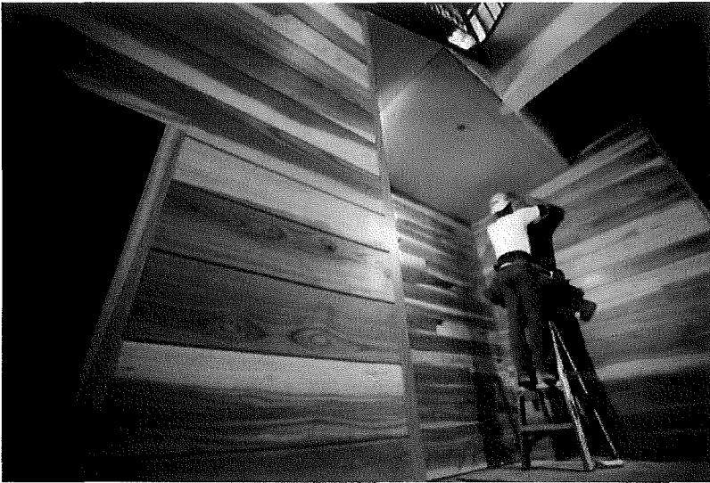
Utilization of wood from felled ash trees in Eagan's Public Safety Center (Photo from Brian Peterson, Star Tribune)
