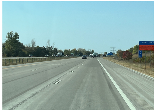
📷 Completed unbonded concrete overlay
