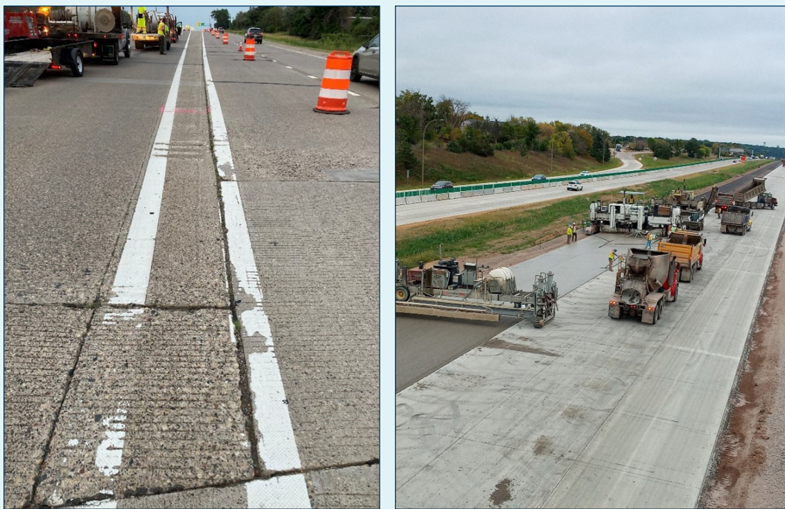
📷 Left image: Roadway before concrete overlay. Right image: Concrete paving. Images courtesy of Robert Golish, MnDOT.
