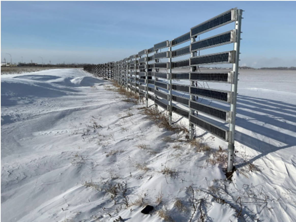
NDSU Solar Snow Fence Photo taken by Dan Gullickson, MnDOT, January 2024.
