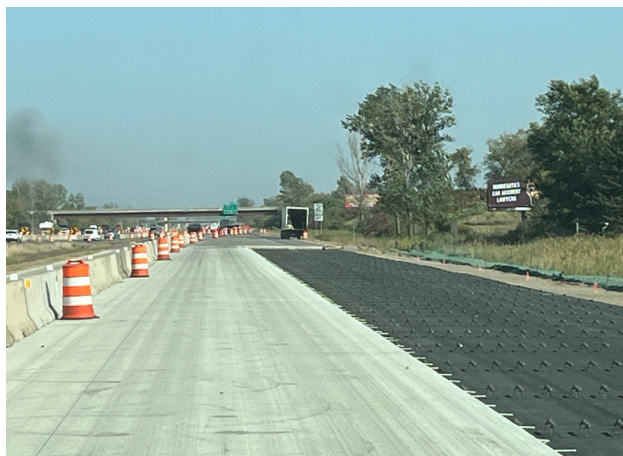
📷 Construction of unbonded overlay
