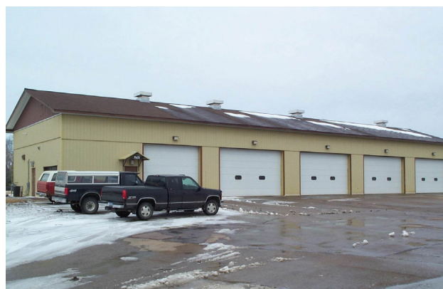
📷 Fairmont truck station, which had an HVAC and Building Automation System (BAS) upgrade in 2023. Photo courtesy of Mark Moehlenbrock, MnDOT.
