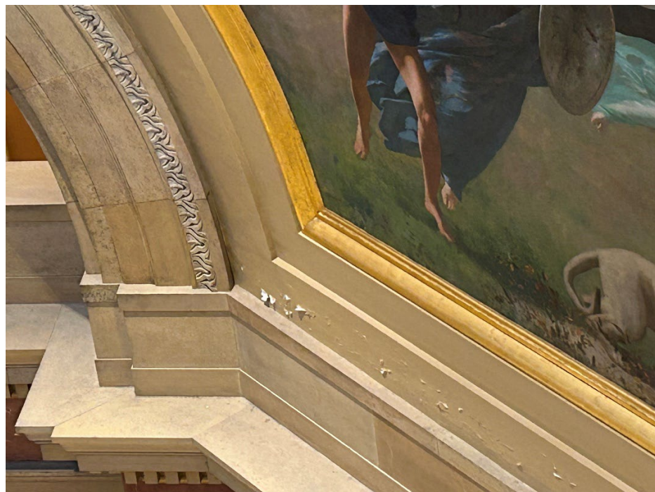
Examples of peeling paint surrounding the fine art in the Capitol Rotunda.
