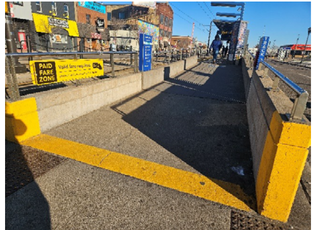
Figure 2b. Photo of paid fare zone sign and boundary line at station platform entrance
