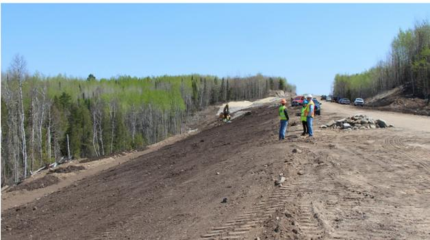
*Roadside soil amended with local industrial by-products can support plant growth and filter stormwater.*
