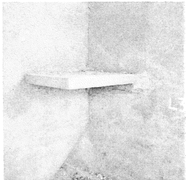
b) Views of 3 1/2 in. x 3 1/2 in. x 3/8 in. bar connectors showing 1/4 in. fillet weld (single side). Figure 4.69. Typical intermediate diaphragm connection.
