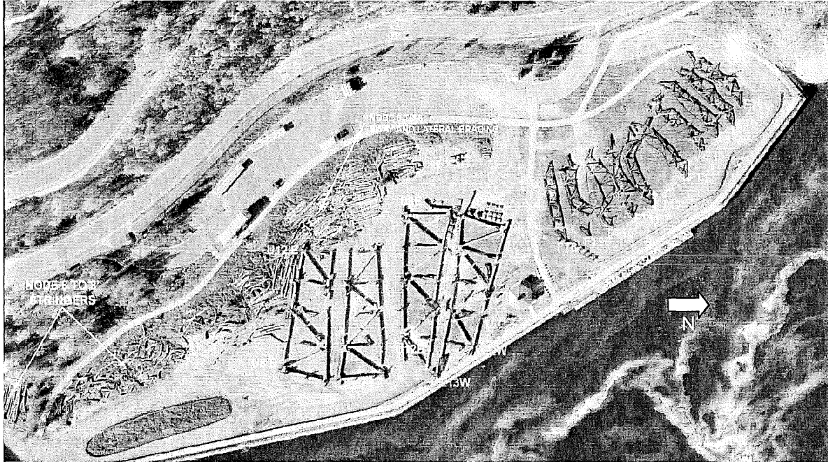
Figure 4.8. Bohemian Flats lay-down site.
