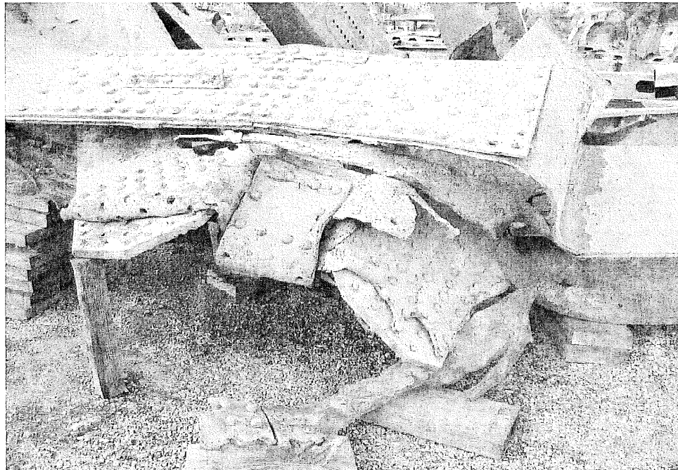
Figure 4.36. L11'W, east elevation facing up.
