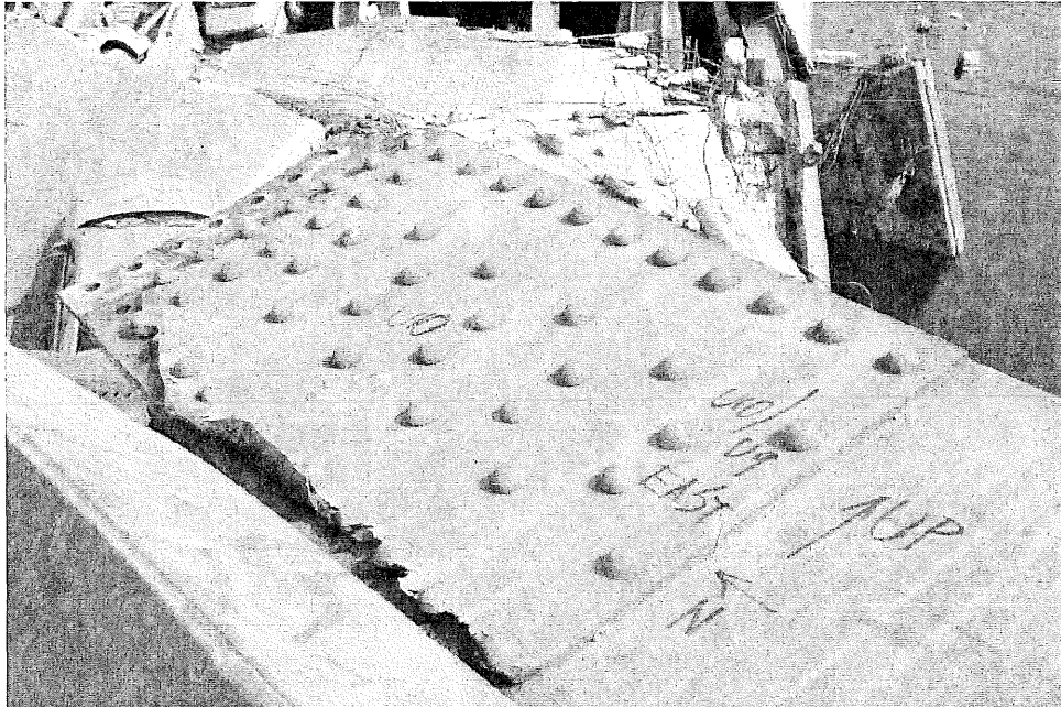
a) West side gusset at U10 end of Upper Chord U9E-U10E
