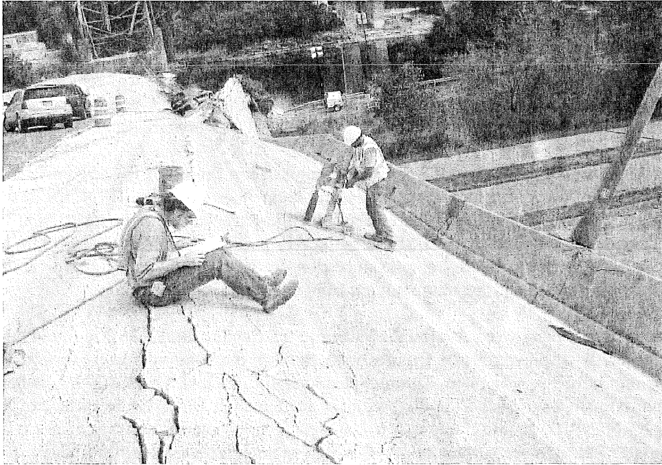
Figure 5.1. Concrete coring of bridge deck.
