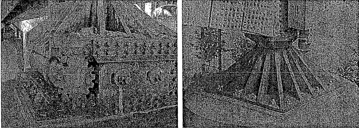
**Figure 2-1. Roller Bearing at Pier 6 (Left) and Fixed Bearing at Pier 7 (Right)**
