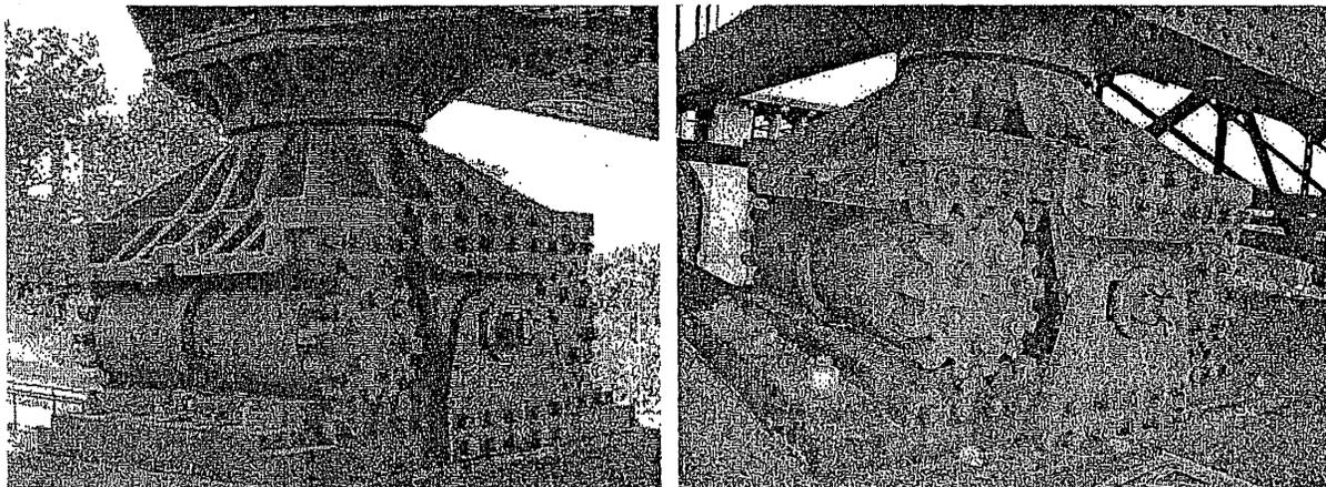
**Figure 2-2. Roller Bearings at Pier 5 (Left) and Pier 8 (Right)**
