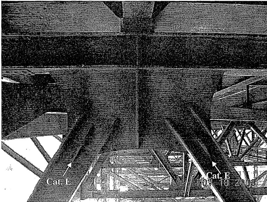
**Figure 1-7. Fatigue Susceptible Details at Floor Truss Joints**
