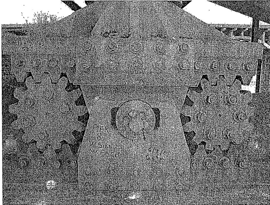
**Figure 2-4. Markings on West Roller Bearing at Pier 8 for Movement Measurement**
