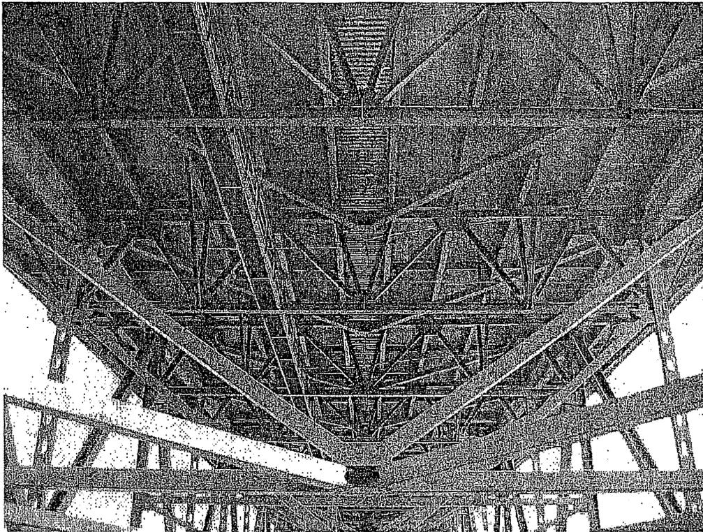
**Figure 3-16: Under Side of Bridge Deck – SIP Forms Between S7 and S8**
