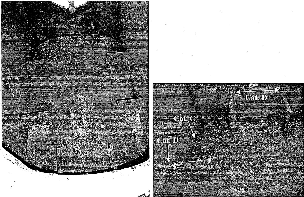
Figure 1-5. Fatigue Susceptible Details inside Main Truss Tension Chords
