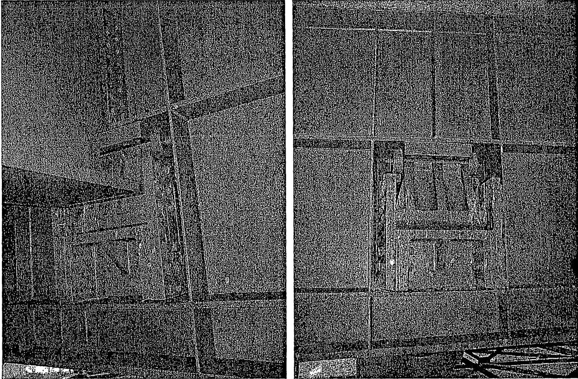
Figure 2-3. Rocker Bearings at North End (Left) and South End (Right) of West Truss
