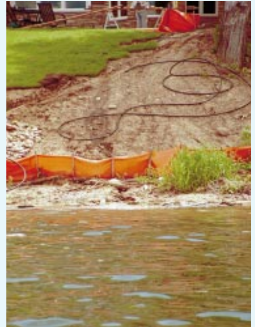
Properly maintained silt fences can minimize erosion caused by construction activities.
