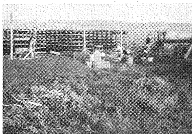
Peat Pellet Pilot Plant in Full Operation. Dried Pellet Stockpile is in Left Center
