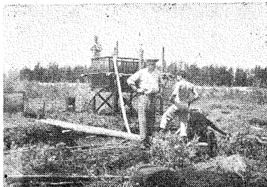
Pumping of Peat Slurry into a Screen Draining Tank
