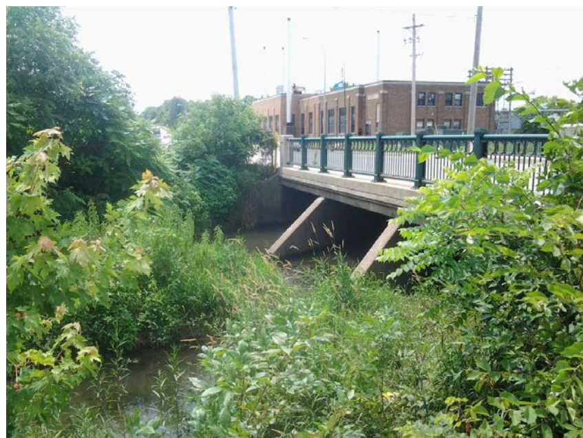
Figure 33: Photo of Culvert 5722, Downstream Side
