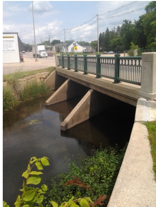
Figure 32: Photo of Culvert 5722, Upstream Side
