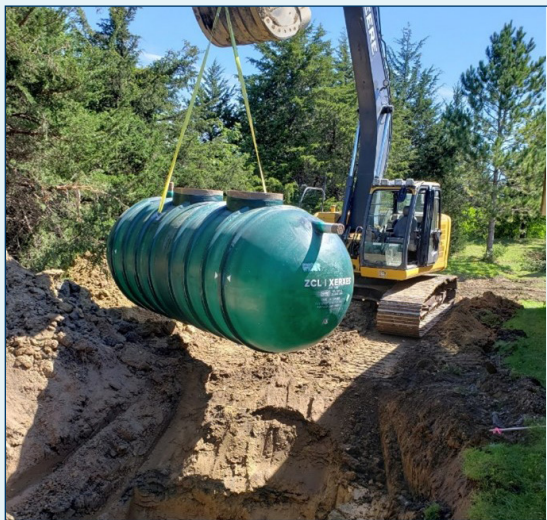
Left: Installation of treatment tank at Buffalo Truck Station. Right: New treatment system in operation at Buffalo Truck Station. Photos courtesy of Neile Reider, MnDOT.
