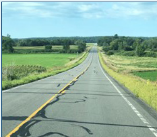
📷 TH 28 before (left) and after (right) the micromill RAP and slurry seal resurfacing project. Photos courtesy of Joel Ulring, MnDOT.
