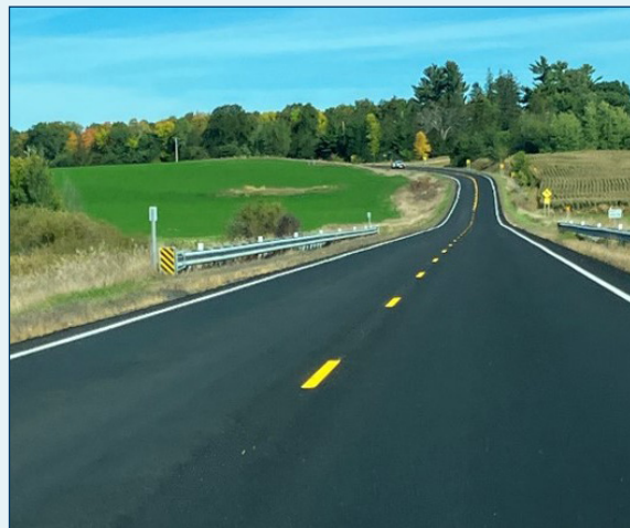
📷 TH 28 before (left) and after (right) the micromill RAP and slurry seal resurfacing project. Photos courtesy of Joel Ulring, MnDOT.
