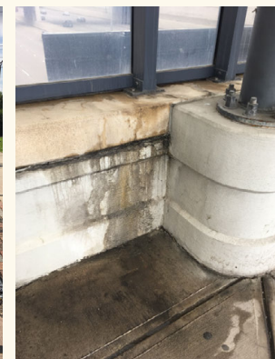
Water damage on Cedar Street Bridge
