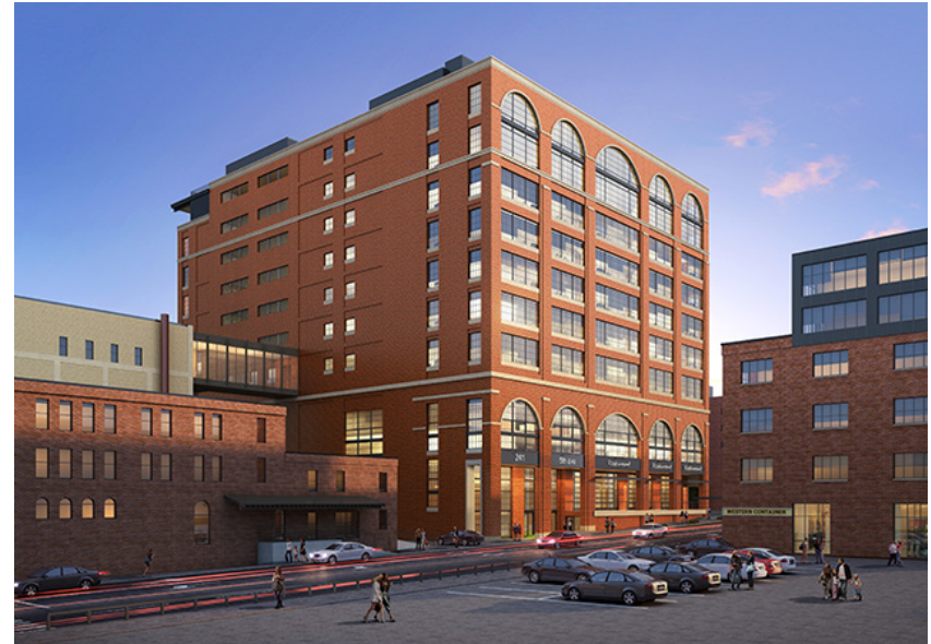
419 Washington in the North Loop, Minneapolis is being developed by Swervo Development and CPM Companies. The building includes three stories of underground parking and five stories of above-ground parking. The building is designed with the capability to convert the parking floors to office space if the parking need goes down. (Image: Courtesy of DJR Architecture)
