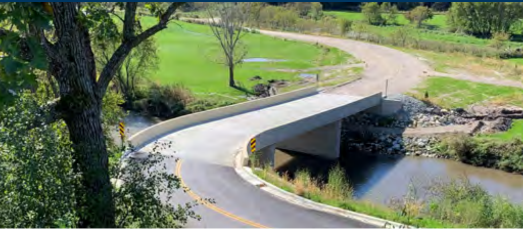
Bridge 23536, Carrolton Township (Fillmore County)
