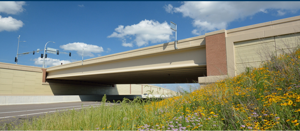
Armstrong Boulevard Bridge (Bridge 02007), City of Ramsey
