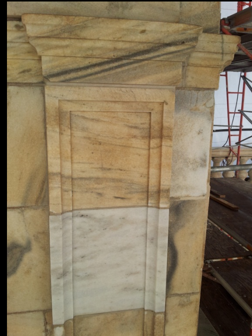
East elevator pilaster - unit replacement 2011
