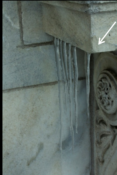
South window hood drip edge (previous patch repair at corner)
