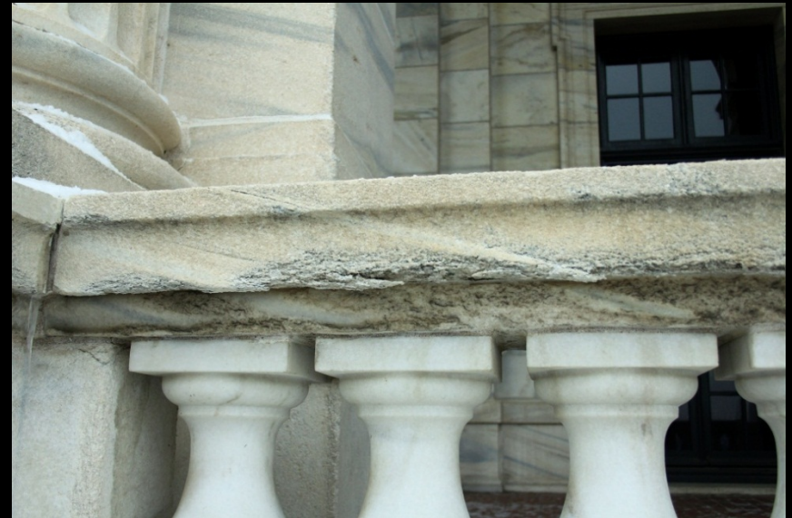
South loggia balustrade rail cap. Balusters were replaced several years ago
