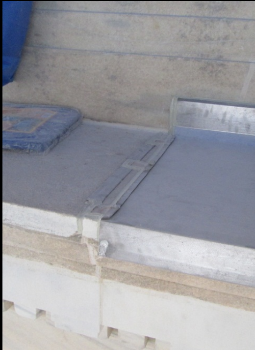
b. Cleats are inserted in joints and flashing is attached to cleats
