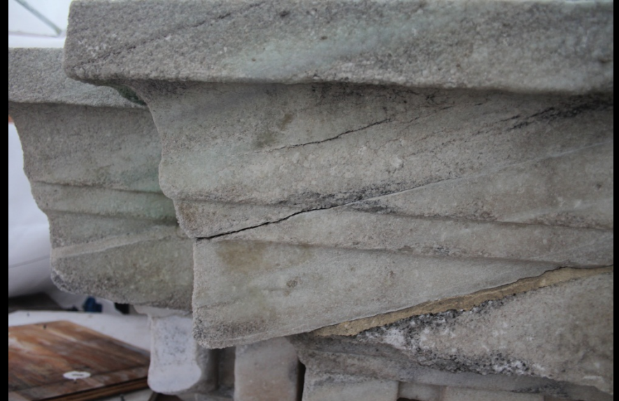
East elevator cornice (side view) – vein erosion and diagonal cracking
