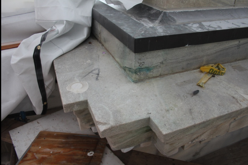
East elevator cornice (top view) – identified in 2010 as possible life safety concern
