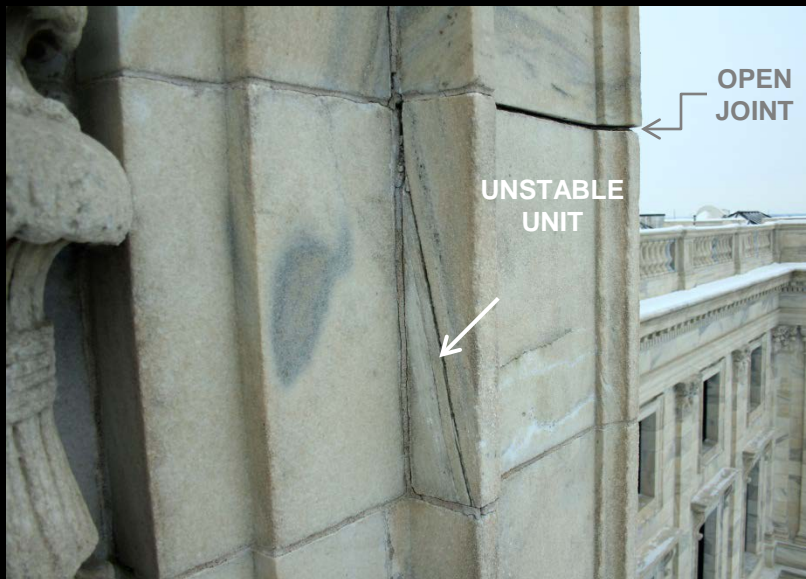
East elevator pilaster (side view) – identified in 2010 as life safety item
