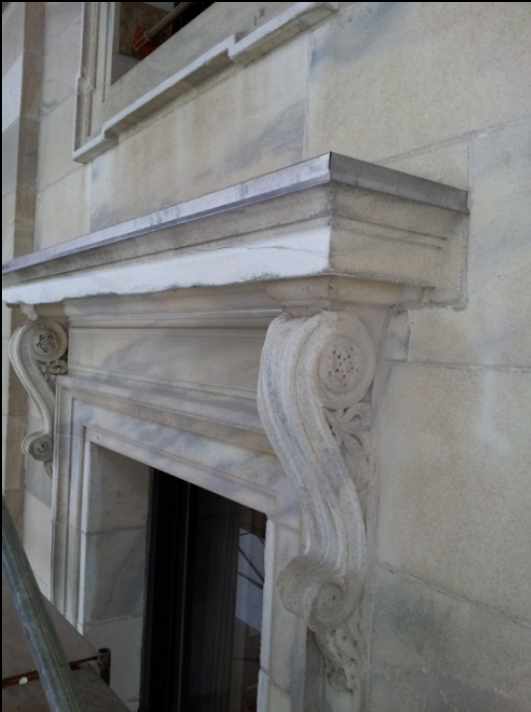
a. Flashing is wrapped and formed over edge of wash ledge to create a friction fit in lieu of fasteners
