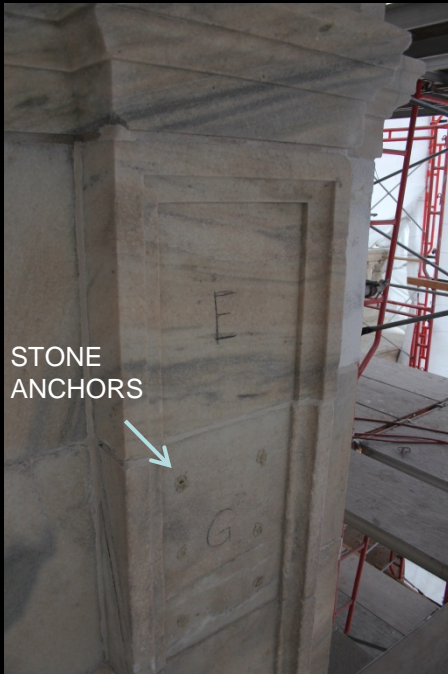
East elevator pilaster– emergency repairs 2010
