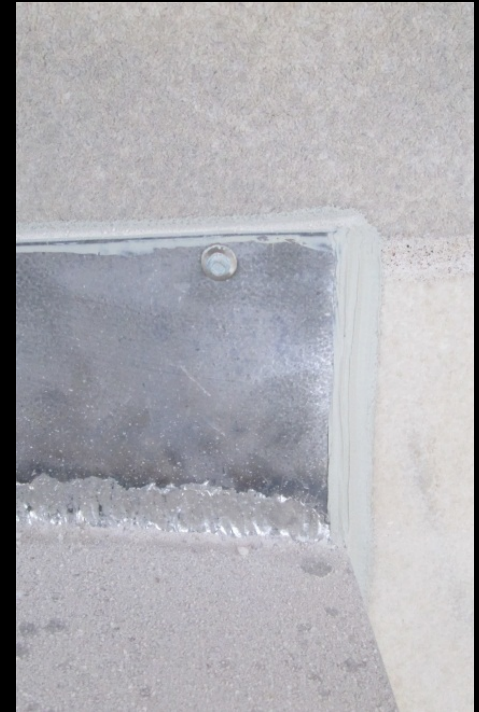
c. Fasteners are inserted in joints. Flashing is custom fit on site to conform to original shape and profile
