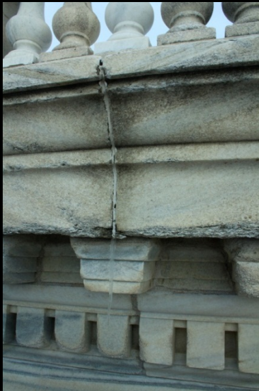
South cornice fascia w/ failed joint
