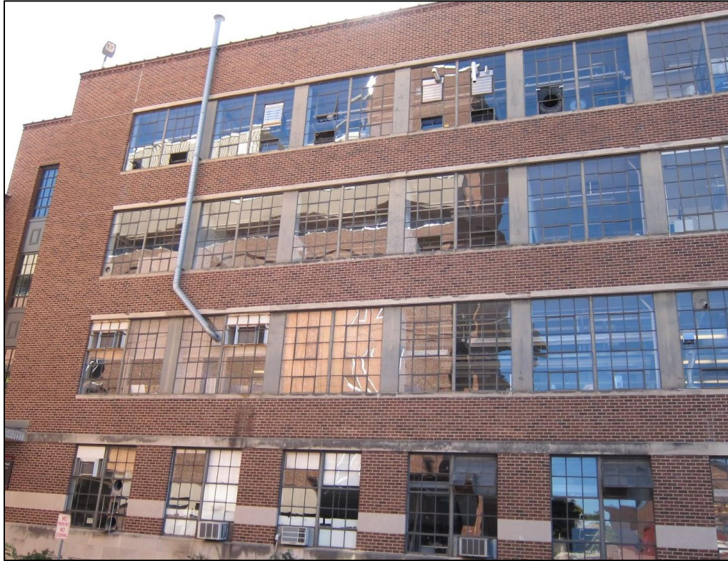
Left: Mechanical Engineering Building; improvised HVAC piping, window A/C units, and makeshift window coverings Right: Typical ab interior pre-renovation
