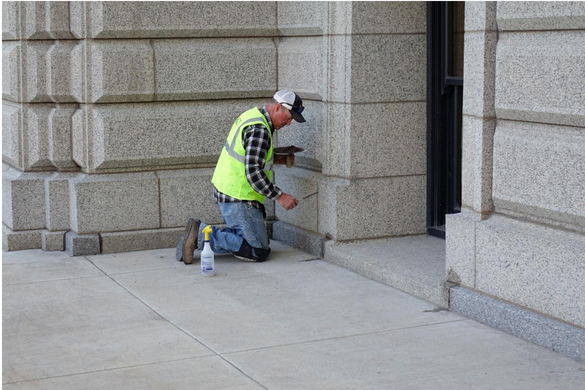
Tuckpoint repair work was performed on the exterior of the Capitol as part of regular, on-going maintenance.
