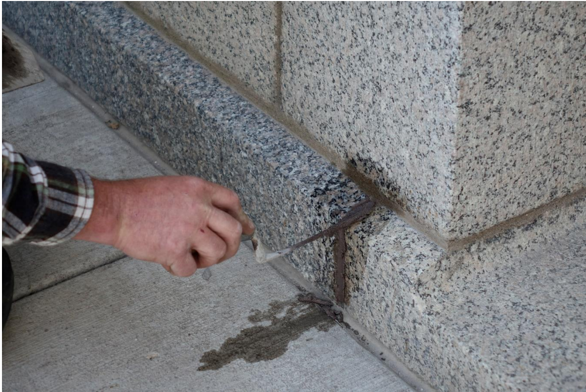
Exterior repair work, such as tuckpointing, on the Minnesota State Capitol requires the expertise and craftsmanship of experienced professionals.
