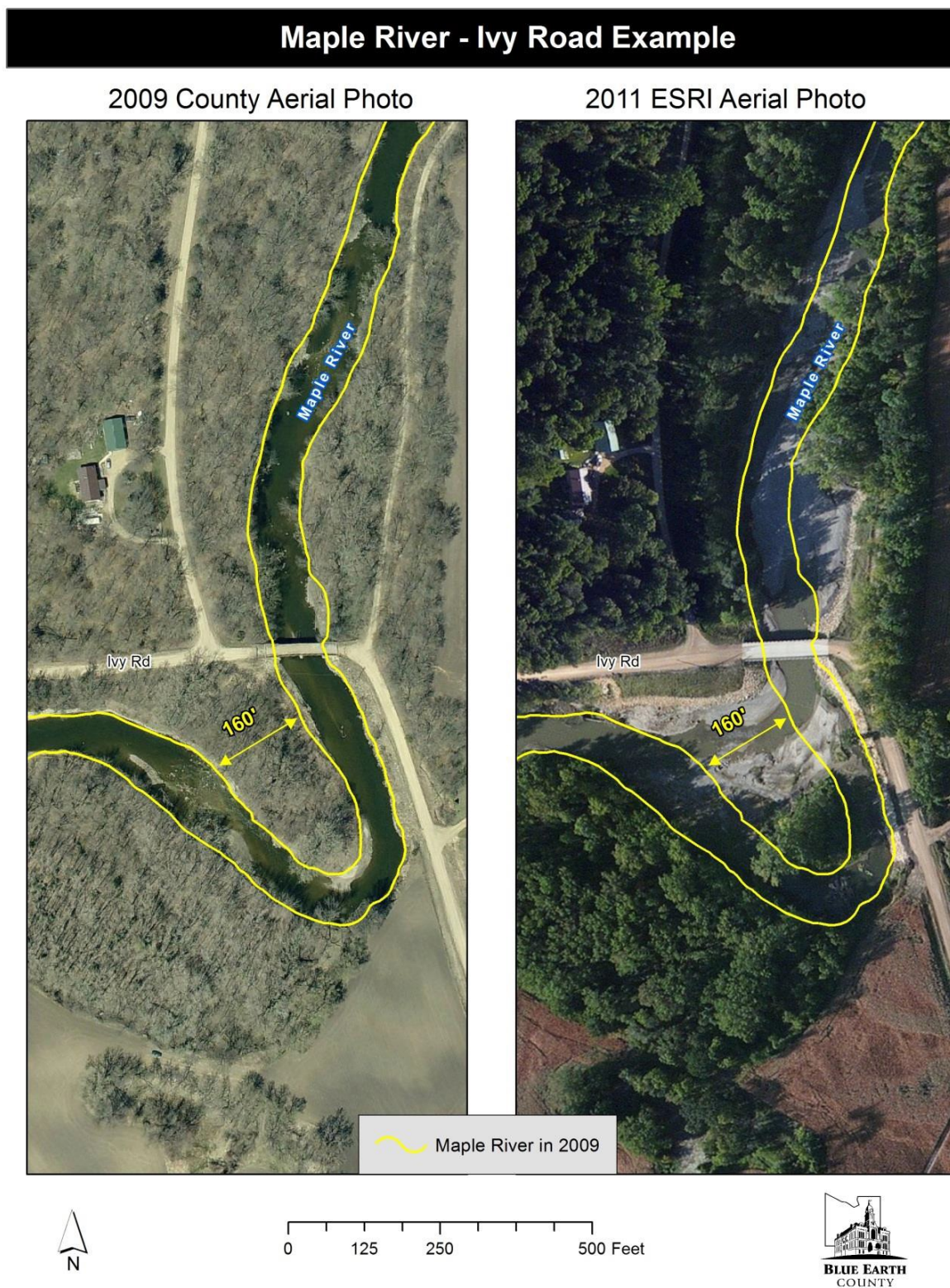
Figure 40 Example of Streambank erosion before event and after restoration, Rapidan Township
