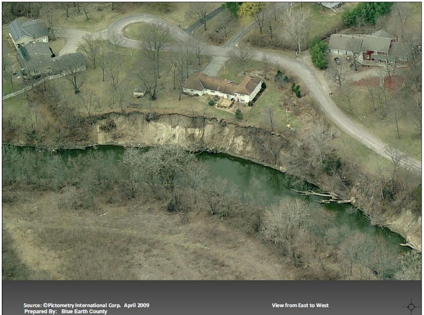
Figure 39 Example of Bluff Erosion
