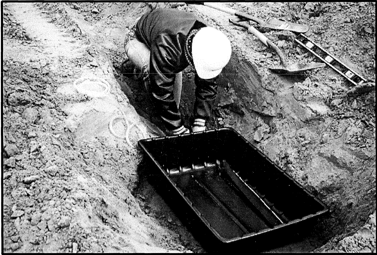
Figure 8. Installation of the lysimeters.
