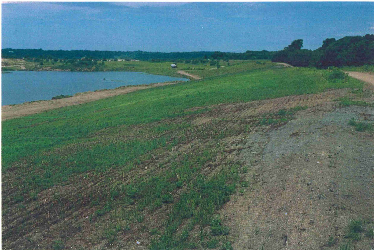
Figure A9.11. Demonstration slope on 7/1/96. With the cover crop (primarily oats) having been almost totally grazed by geese, the plants seen in this photo are mostly ragweed and lambsquarter.
