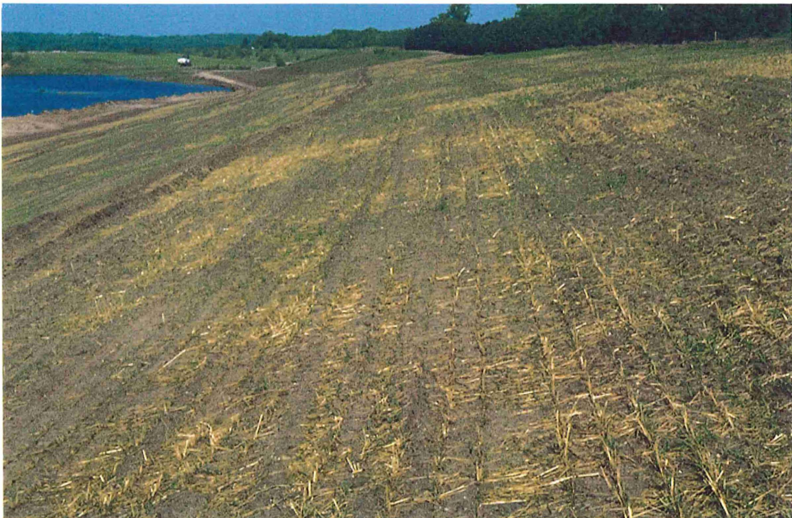
Figure A9.10. Crimped-in mulch, as seen two weeks after mulching was completed. Note the lack of mulch in the lower left hand corner, typical of the open areas that remained after mulching.
