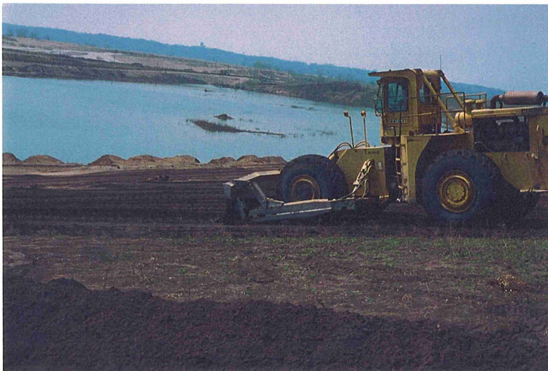
Figure A9.4. Filling in erosion gullies and spreading topsoil prior to amendment spreading.
