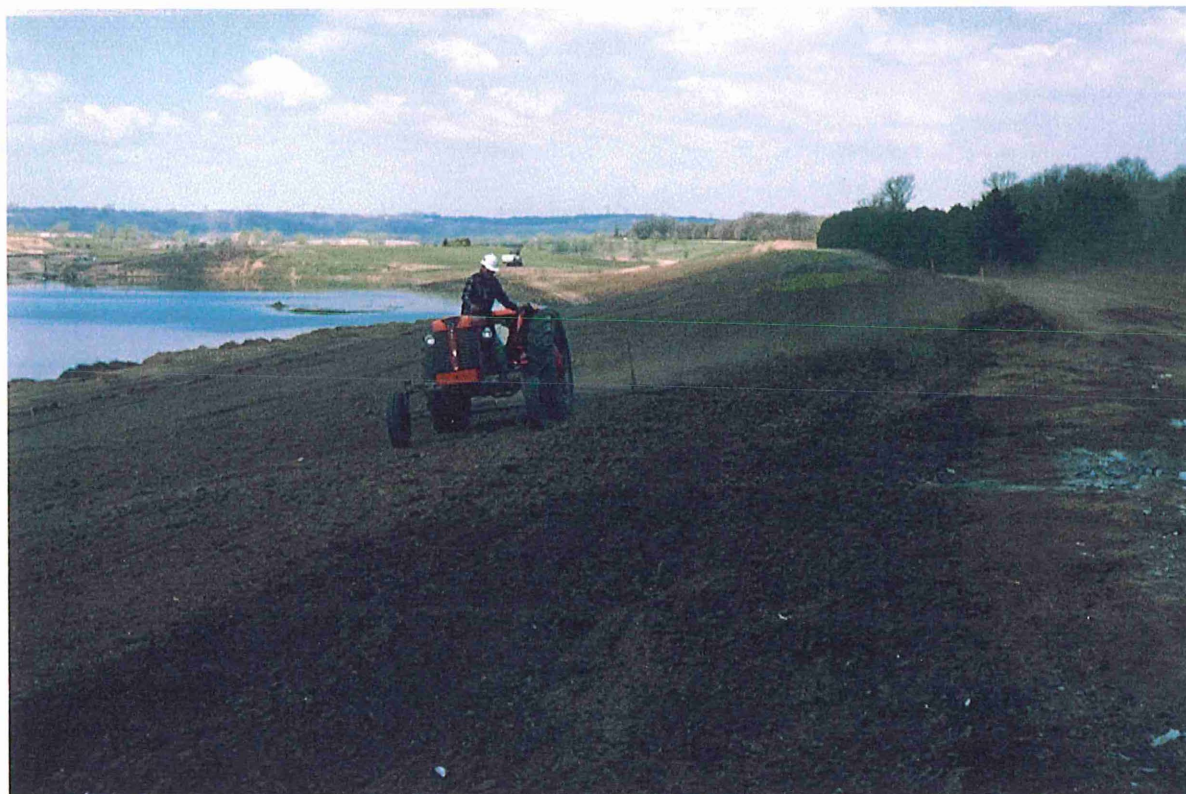
Figure A9.7. Seeding the upper third of the plot with the MNDOT 50A seed mix.
