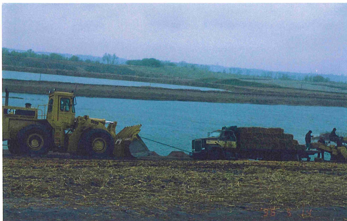
Figure A9.8. Mulching the demonstration slope with a platform-mounted blower. The truck with the hay bales was unable to maneuver on the sandy slope, so the front-end loader was brought in to pull the truck and blower. This produced depressions in the slope, as well as compaction.
