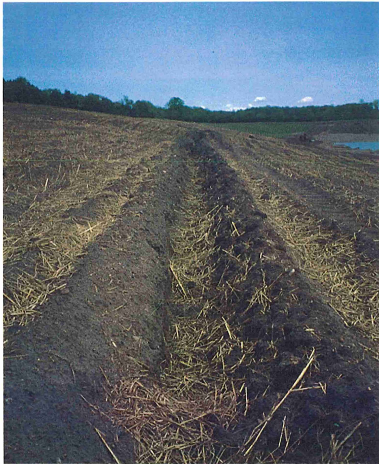
Figure A9.9. One of the two trenches that run across the width of the demonstration slope, as seen after mulching was completed.
