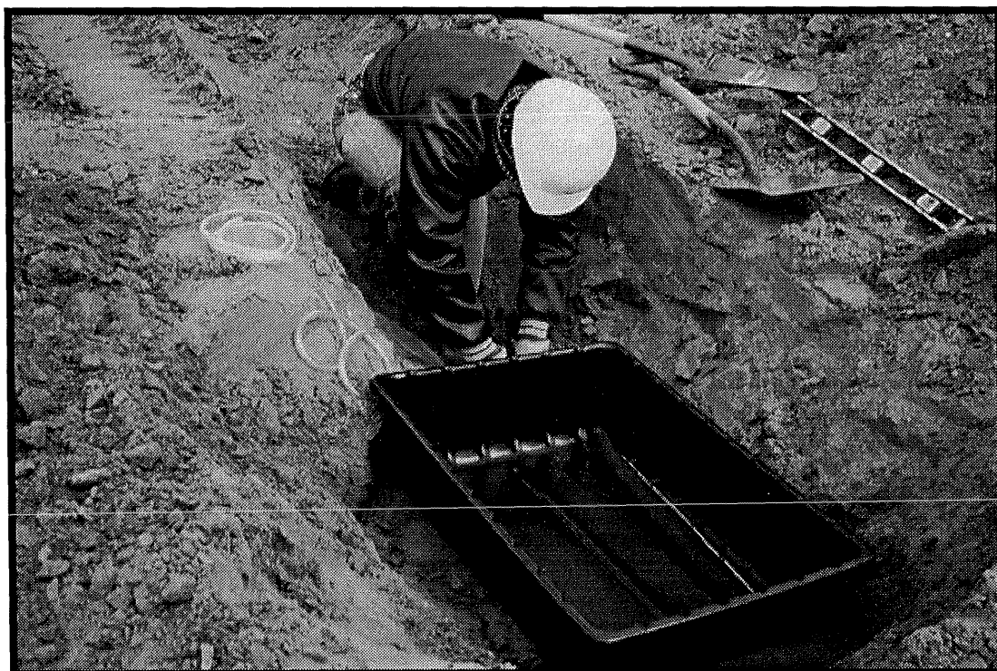
Figure 7. Lysimeter installation.
